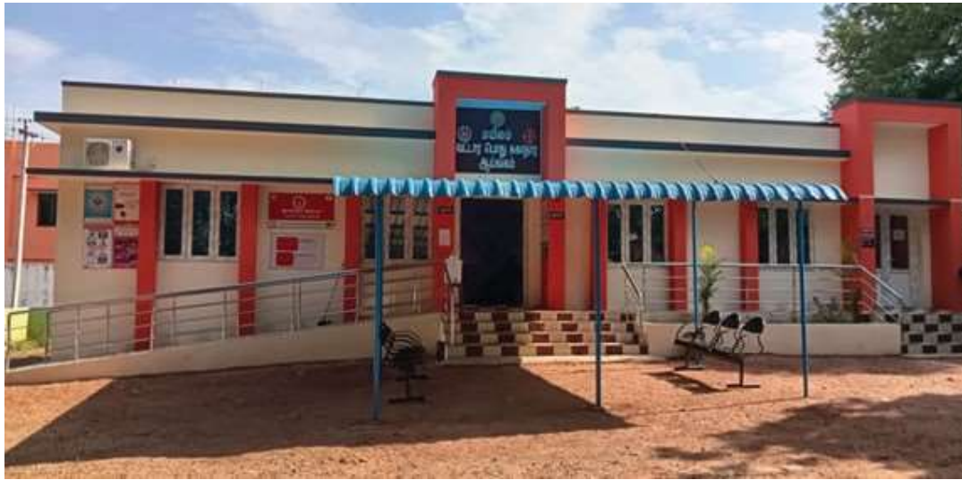
Figure 3.4: New building for laboratory services and Office Administration in an accredited primary facility
